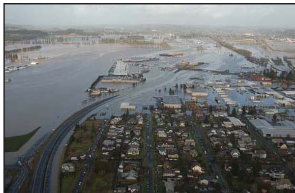
Flooding on I-5 in Lewis County
